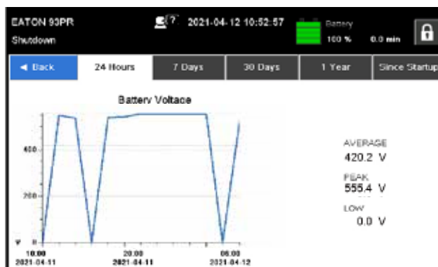
Figure 6-17: Battery Voltage Screens
